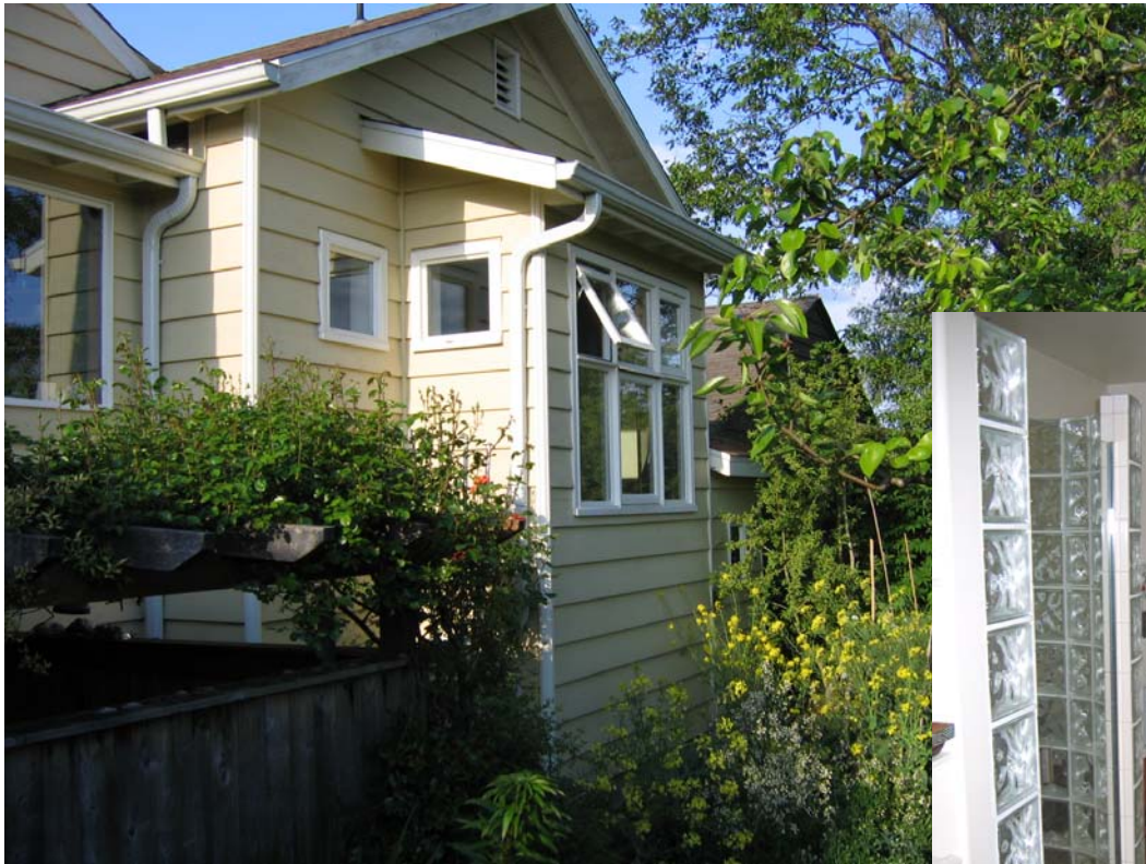
The addition looks over a lush backyard garden
